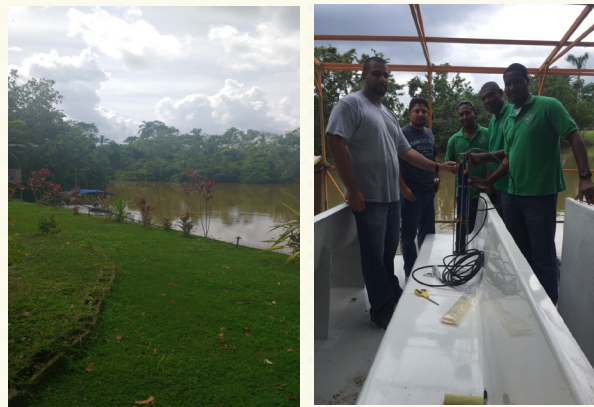
Installation of second sonde near Burrell Boom Village
