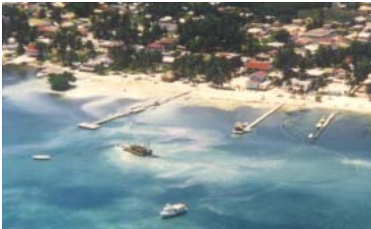
Dredger pumping sand on land for Caye Caulker beach replenishment (CZMAI)
