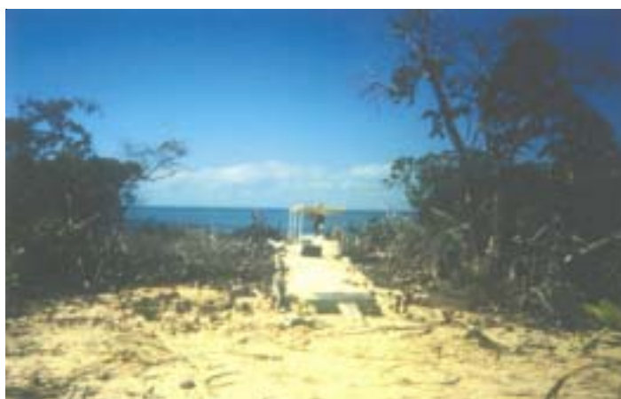
Mangrove cleared to allow for pier construction (CZMAI)
