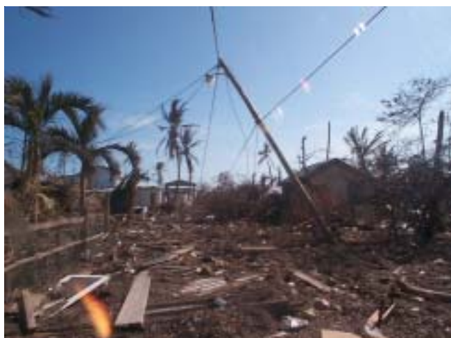
Destroyed and damaged infrastructure on Caye Caulker following Hurricane Keith. (CZMAI)
