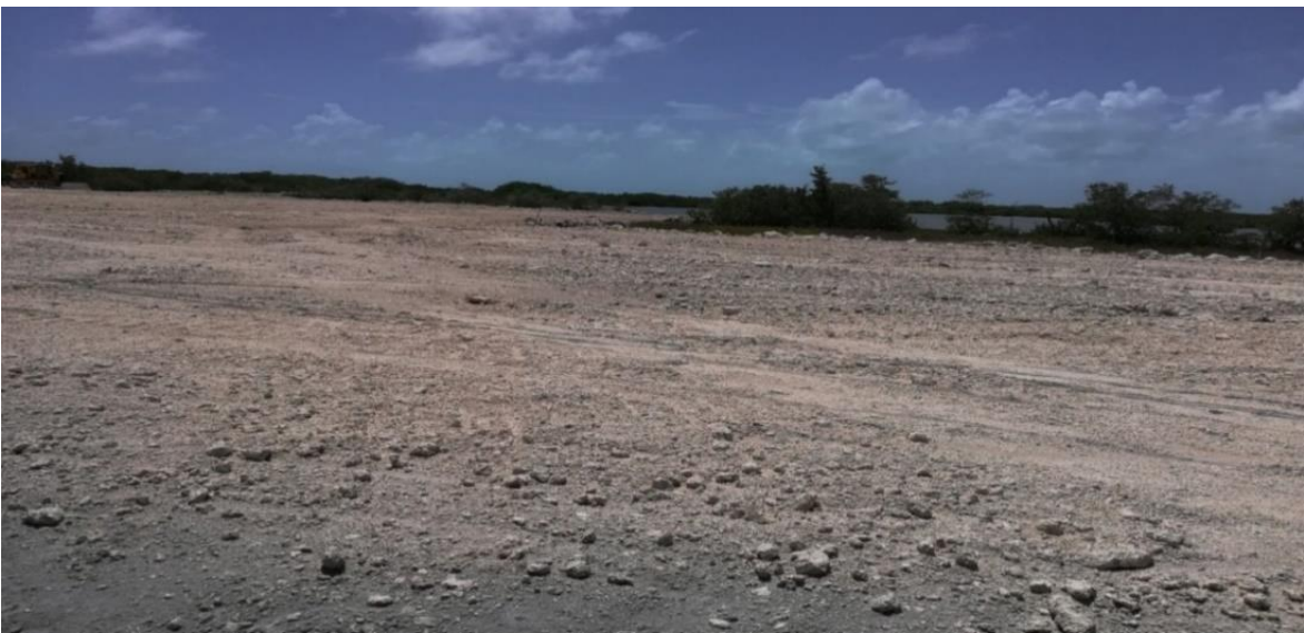
Figure 16 Proper landfill of mangrove swamps with stones and sand
