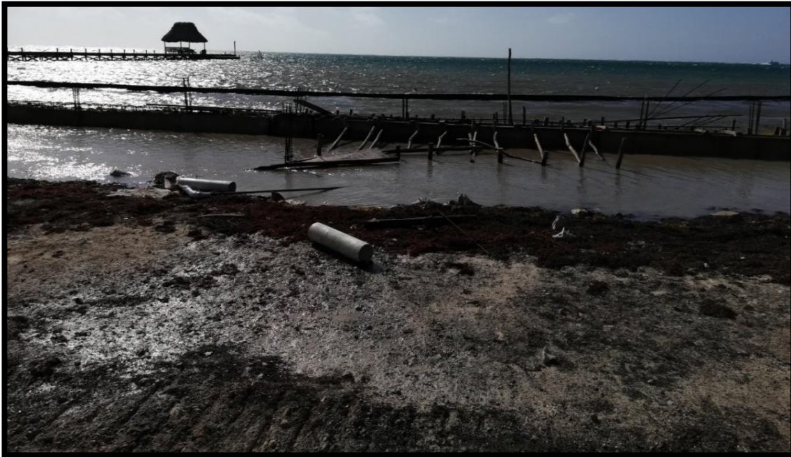
Figure 11 Erection of defence structure to reclaim land and stop erosion
